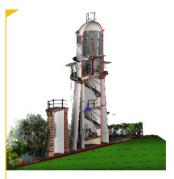
Our first Heritage Information Modelling project, the Green Island Lighthouse Compound is an exemplary use of Laser Scanning, Drone Photogrammetry, BIM and Asset Data collection and storage. Each element is highly detailed and hosting data about the object and its historical significance.
